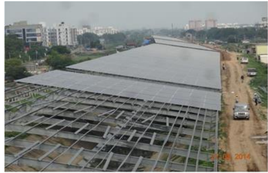
Figure 3. New Sama steel truss structure
