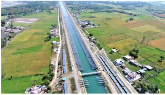
Figure 5. Suspension cable structures on Yamunua Canal
