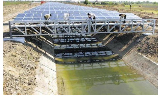
Figure 2. Pilot plant steel truss structure
